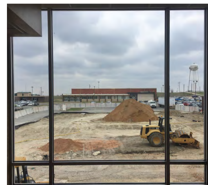
Zachary Pletan’s photo of Grayson’s progressing construction
